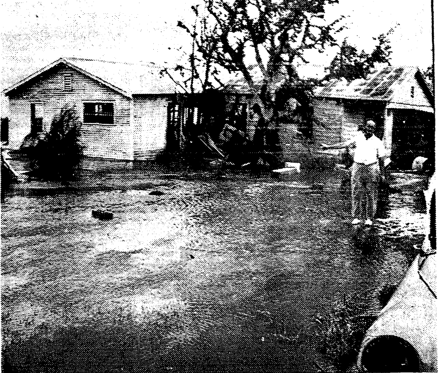
—Photo by The Times-Picayune. STANDING by a relative's house in Delacroix Tuesday afternoon is E. T. "Tom" Treadaway, who said the waters surrounding the house battered by Hurricane Betsy rose with the approach of tropical storm Debbie Tuesday. The area had drained since Betsy's visit and the house was on dry ground, he said. He also said that only six out of 300 houses in Delacroix withstood Hurricane Betsy. (Map in Sec. 1, Page 3. Other Pictures in Sec. 3, Page 20.)
