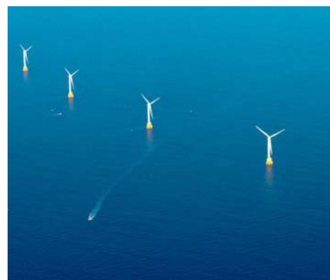
The first U.S. off shore wind farm, built off Block Island, R.I. in 2016.
